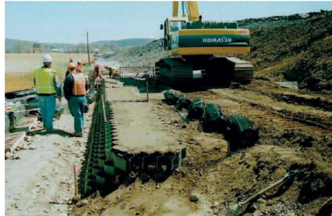
Photo 2. Today's geocell mats expand to form "honeycombs."
