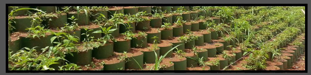
A gravity wall must be able to hold together as a unit in order to function. It must be stable in respect to both external forces that would cause it to fall as well as internal forces that could cause deformity or loss of shape.
